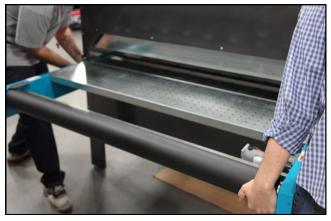
2. With another person and two flanged nuts in hand, lift up the outfeed and insert it into the four exposed hex bolts.
